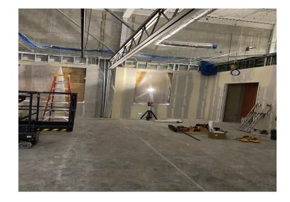
KWIK-SPAN – Select Kwik-Span if the partition's location cannot be accessed easily with up to 21 ft. long Unispan truss sections eg: a high-rise commercial building above the ground floor or where exterior window removal and re-install is cost-prohibitive. Kwik-Span is fully assembled at the partition's location and Kwik-Span component parts can easily be transported in a building's service elevator.
